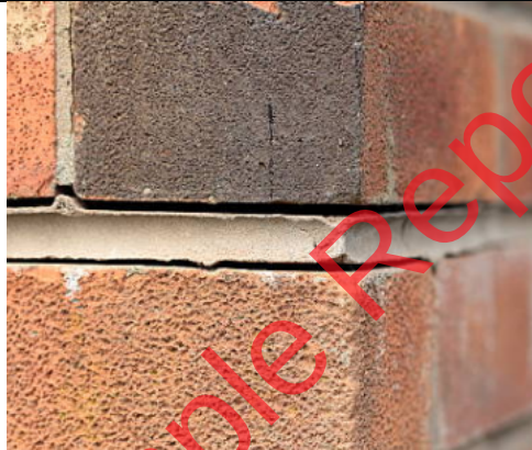
Isolated detached mortar
