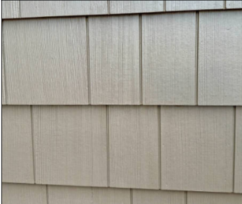
Shingle style composite siding in very good condition
