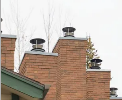
Typical metal chimney caps
