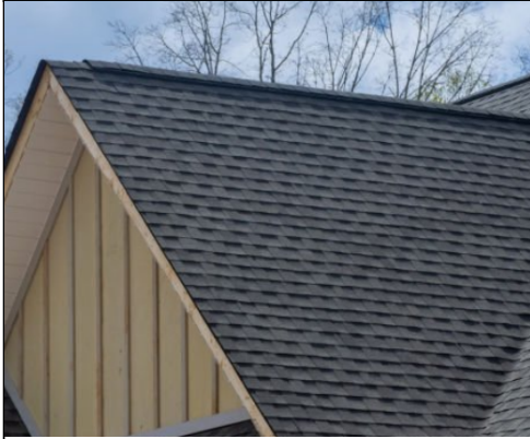
Asphalt shingle roof with ridge vent
