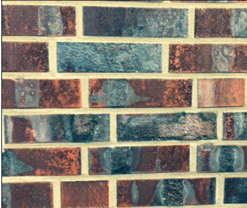
Mortar joints in good condition
