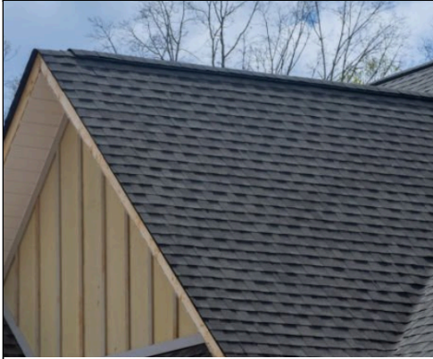
Asphalt shingle roof with ridge vent
