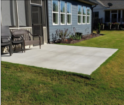
Typical concrete patio
