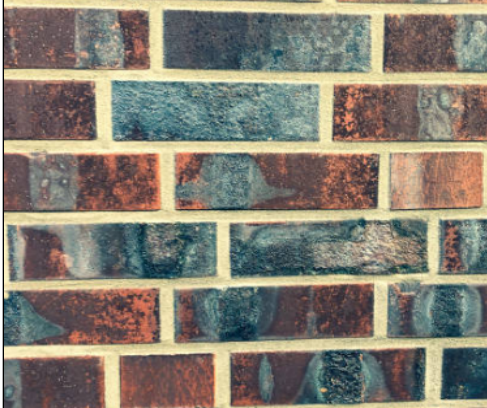
Mortar joints in good condition
