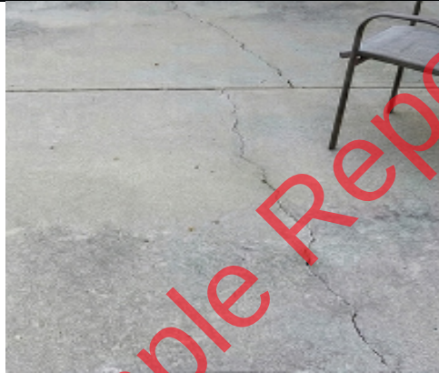
Concrete cracks
