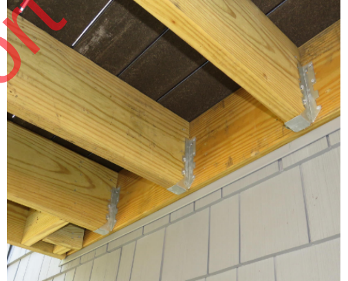
Wood joists with metal hangers
